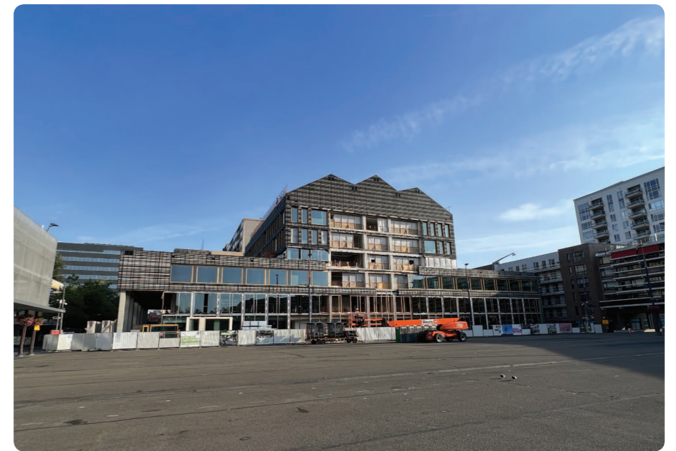
September 2022 - start montage Fraké houten latten
