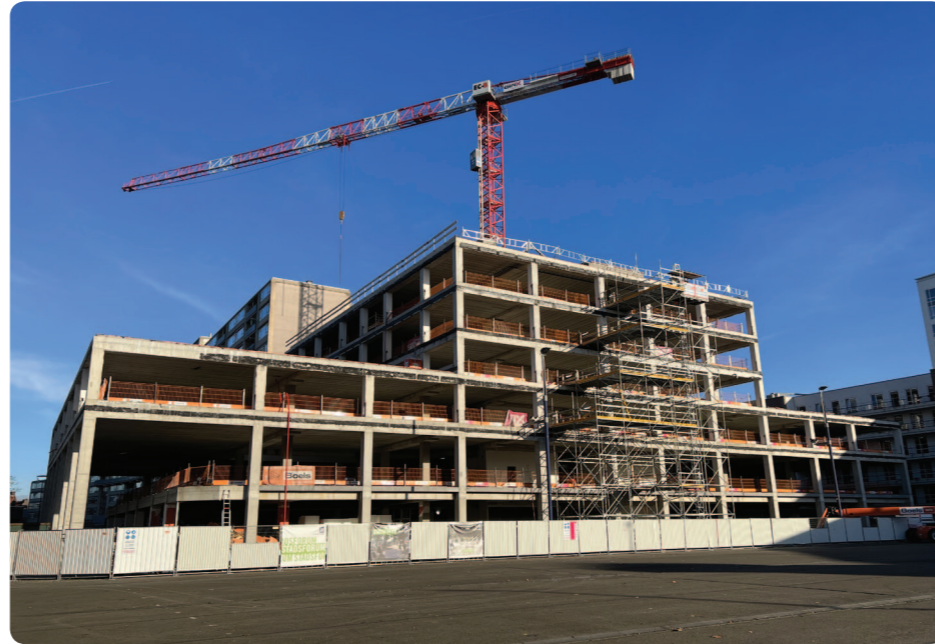
September 2021 - sloop gereed
