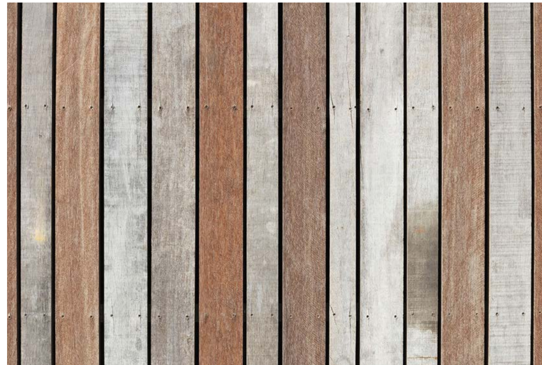
reclaimed wood as facade cladding (wood formerly used as quay wall protection)
