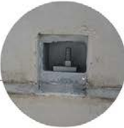
DEMOUNTABLE STRUCTURE in precast concrete
