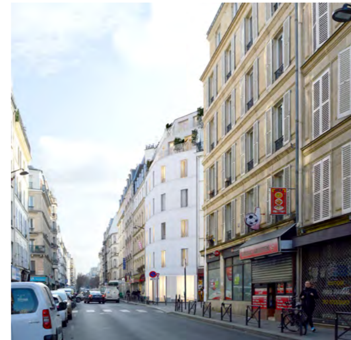
Paris 17th district Beginning of renovation and extension of a hotel and housing.
