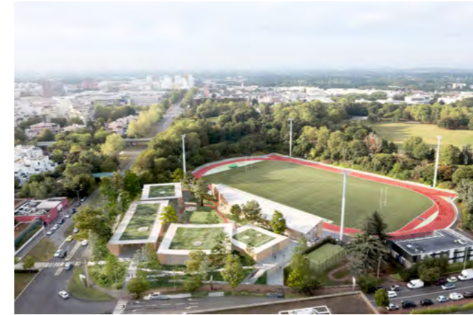
Evry-Courcouronnes Children's center, sports equipment and 300-seat grandstand.
