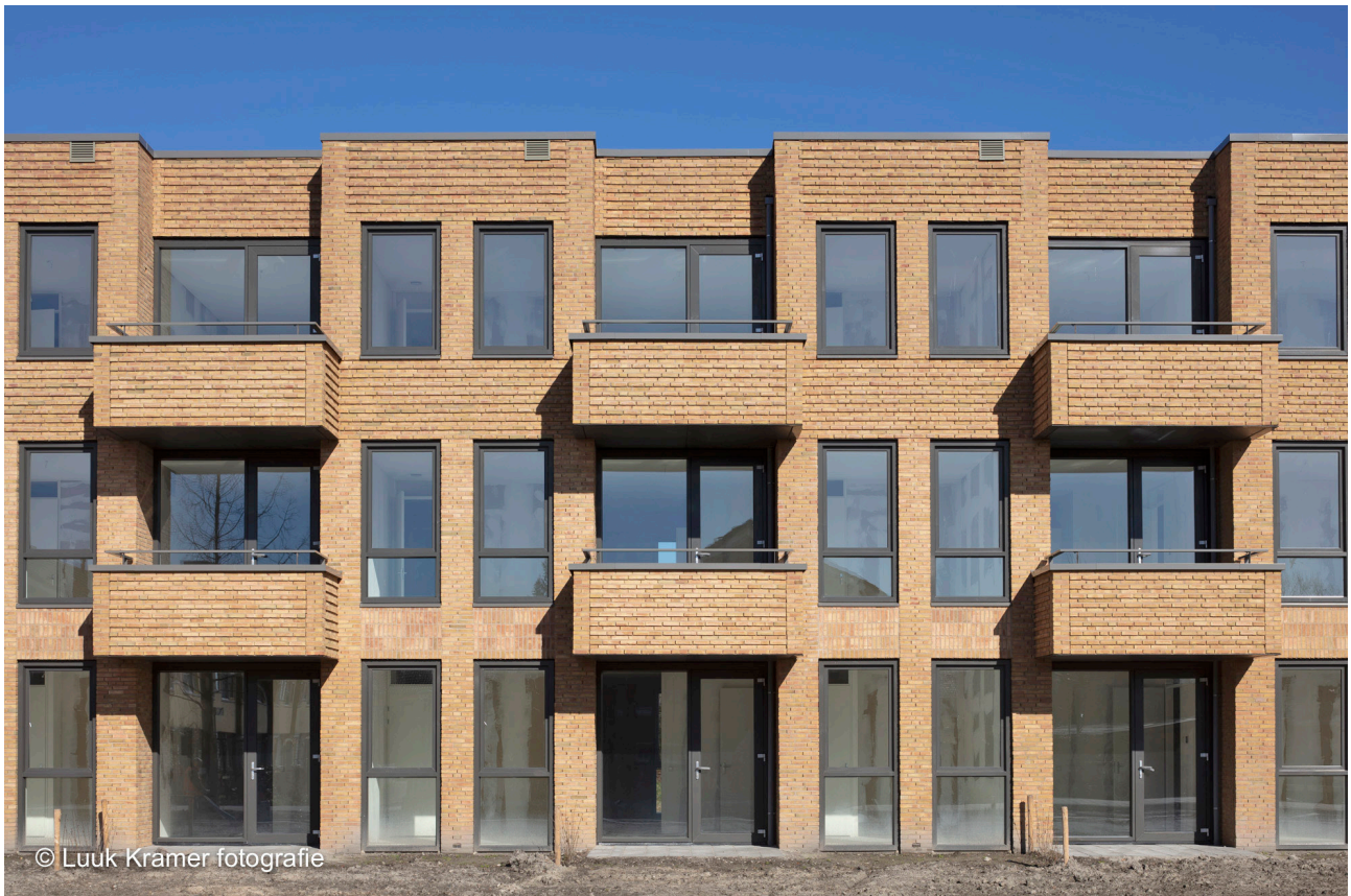
Facade fragment courtyard-side
