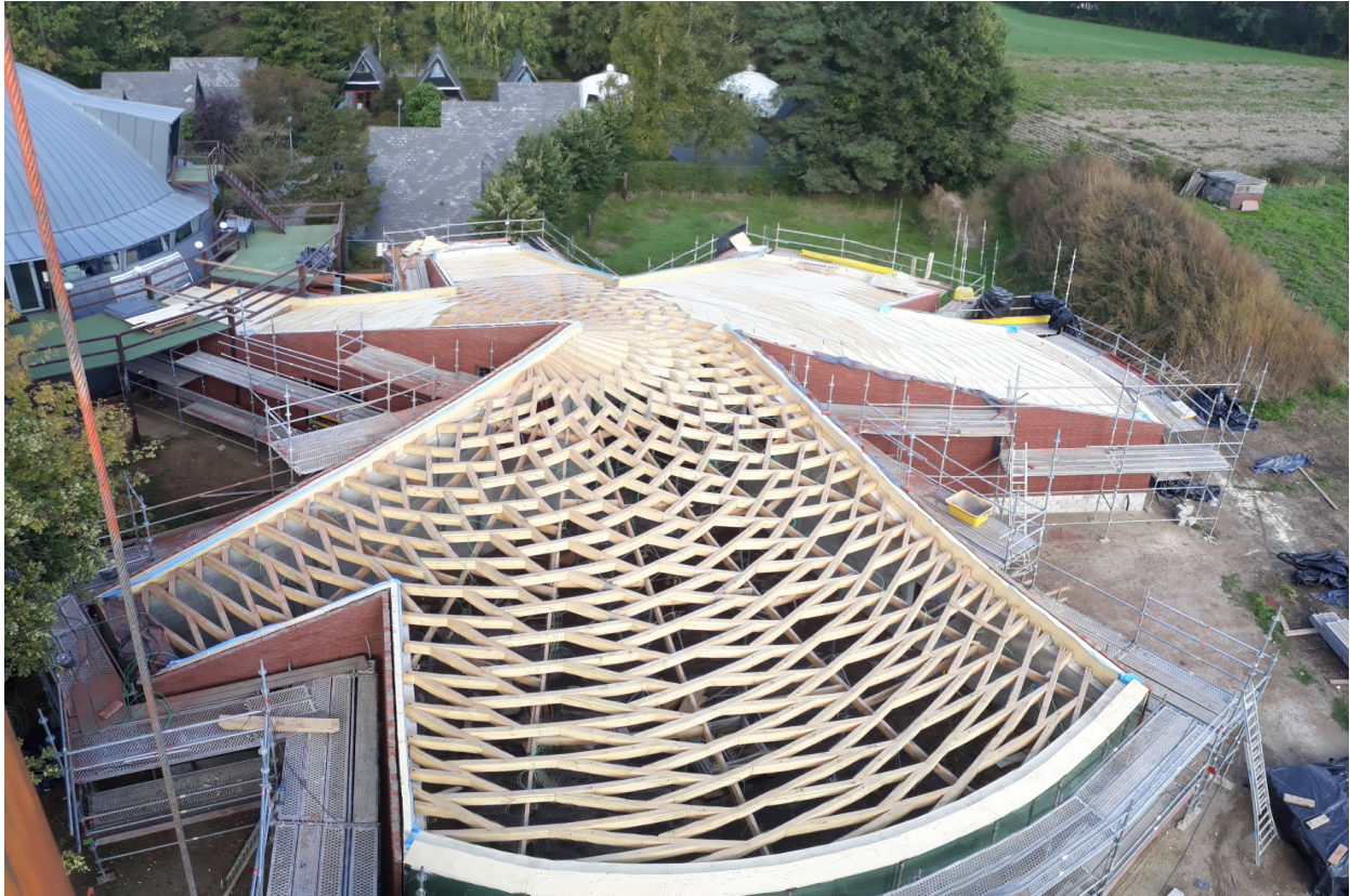
Aerial view of the new pavilion during construction (© photography Vanhout Pro)
