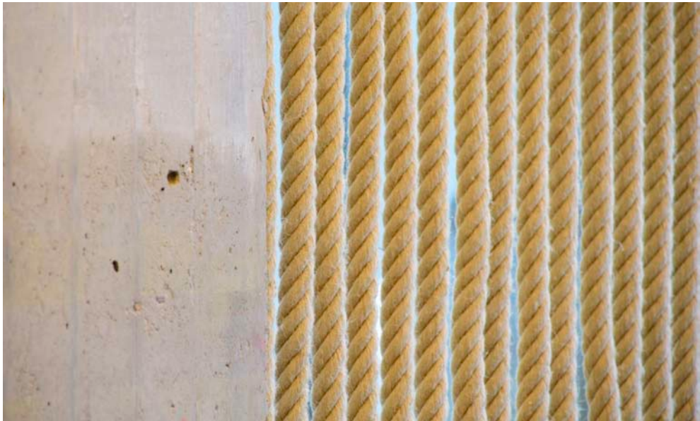
Detailfotos: Akoestische leren achterwand met ingestikt logo van Vesteda en akoestische privacyschermen van touw. Details: Akoestic leather wall with stitched logo and ropes that are used as privacy screen with akoestic performances.
