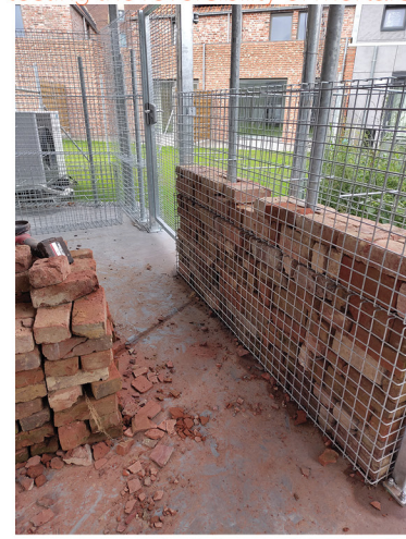
building gabion walls
