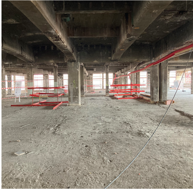
Heavy concrete beams and columns on level +1, with limited free height
