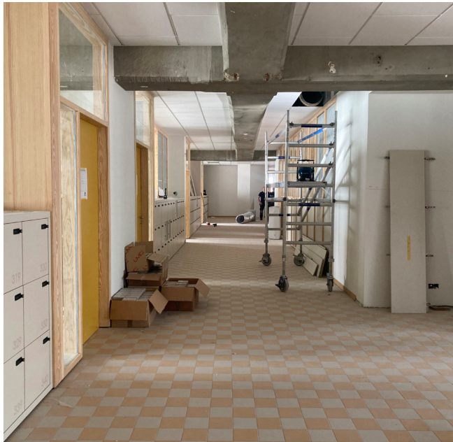
New classrooms with existing structure visible
