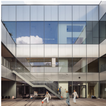
New patio in existing building for daylight and access
