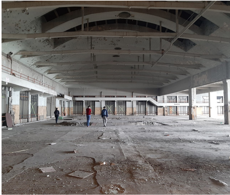
Former bottling plant with characteristic vaulted roof, before start of construction
